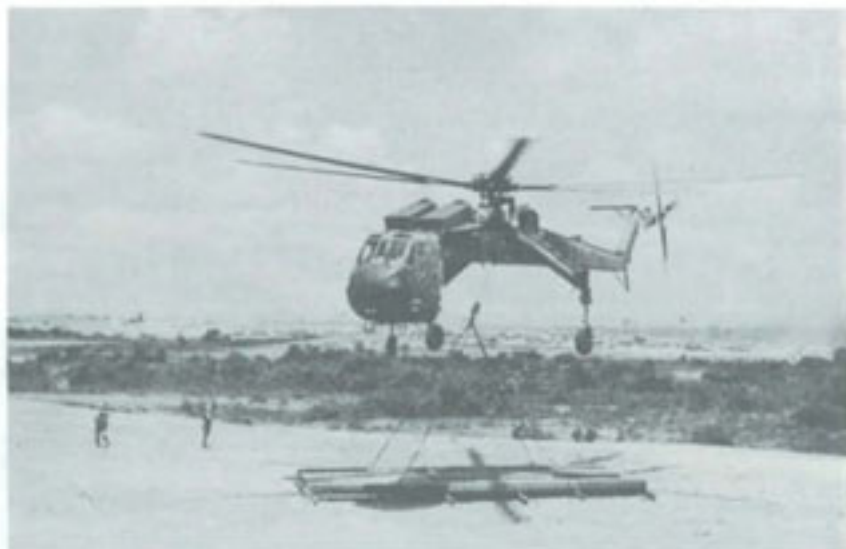
SKY CRANE LIFTING BRIDGE SPAN
