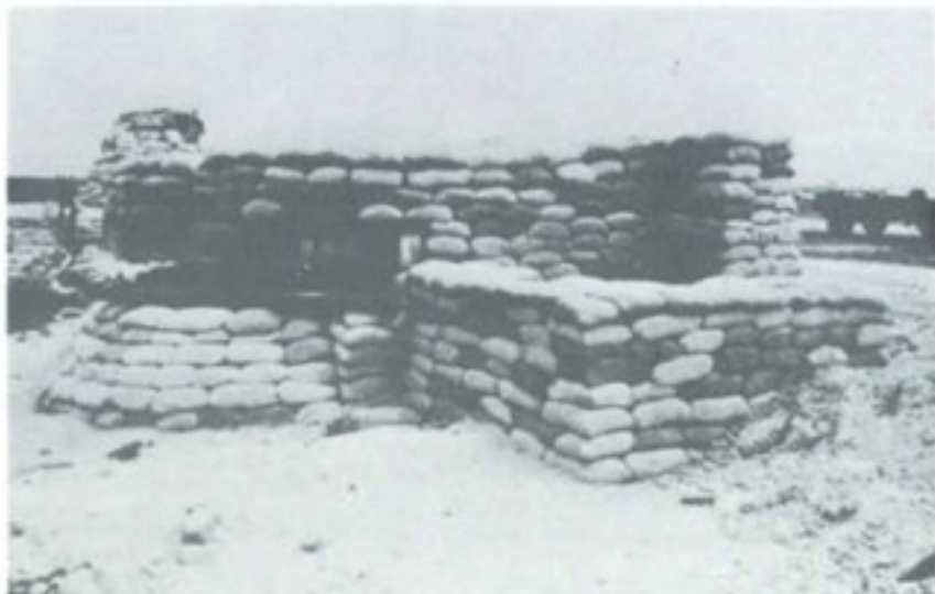
SANDBAG-REVETTED MACHINE GUN POSITION AT DAU TIENG
