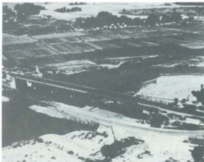
PERMANENT BRIDGE ON HIGHWAY 19 BETWEEN QUI NHON AND AN KHE replaces tactical one-lane Bailey bridge.
