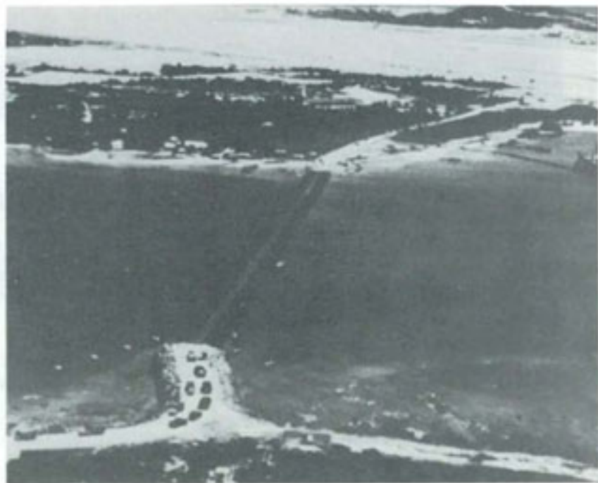
AERIAL VIEW OF MY CA FLOAT BRIDGE, with 10,000-foot Cam Ranh airfield runway in background. Radio-connected control points at each terminus directed traffic.
