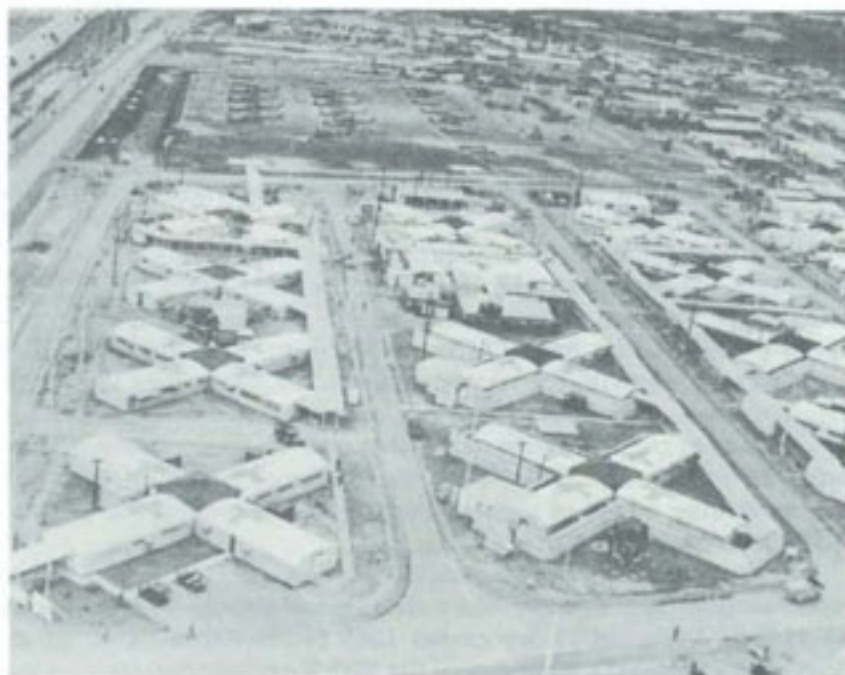
THE 93D EVACUATION HOSPITAL AT LONG BINH. In an advanced state of construction in the spring of 1966 and of unique local design, this hospital had revetments around critical wards and on two sides of helicopter barking stands. Blackened area was treated with dust palliative.
