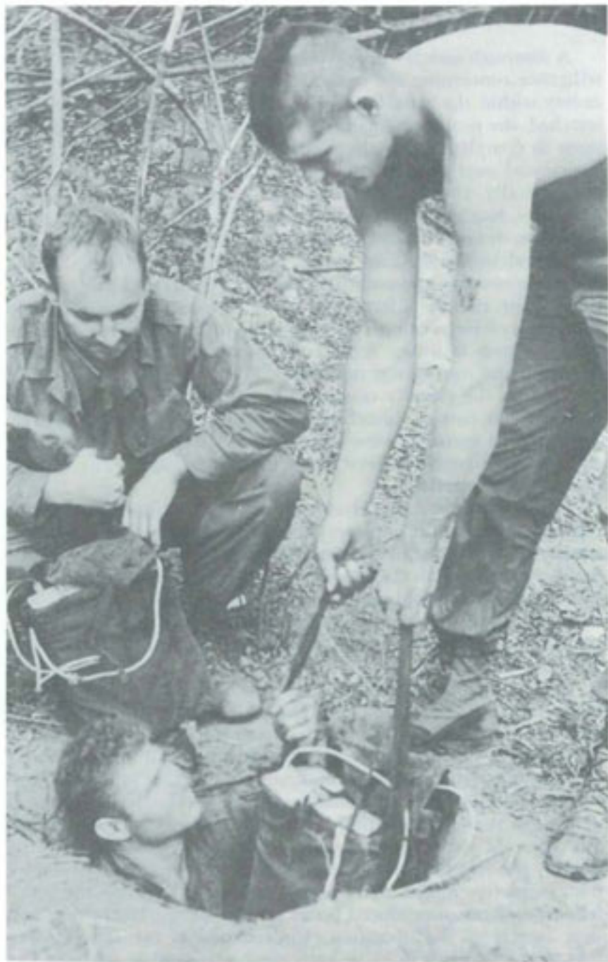
ENGINEER TUNNEL DEMOLITION TEAM. "Tunnel rat" is preparing to place charges and make connections for detonation. Note smallness of access hole which is easily camouflaged.
