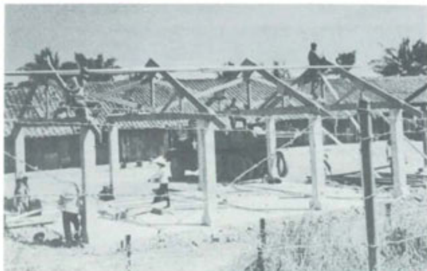
VILLAGERS AND ENGINEERS CONSTRUCT PUBLIC FISH MARKET AT RACH KIEN
