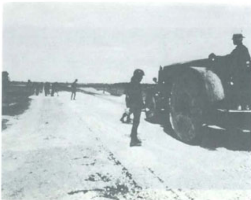
VIETNAMESE ENGINEERS WORKING ON HIGHWAY 9 NEAR DUC HOA
