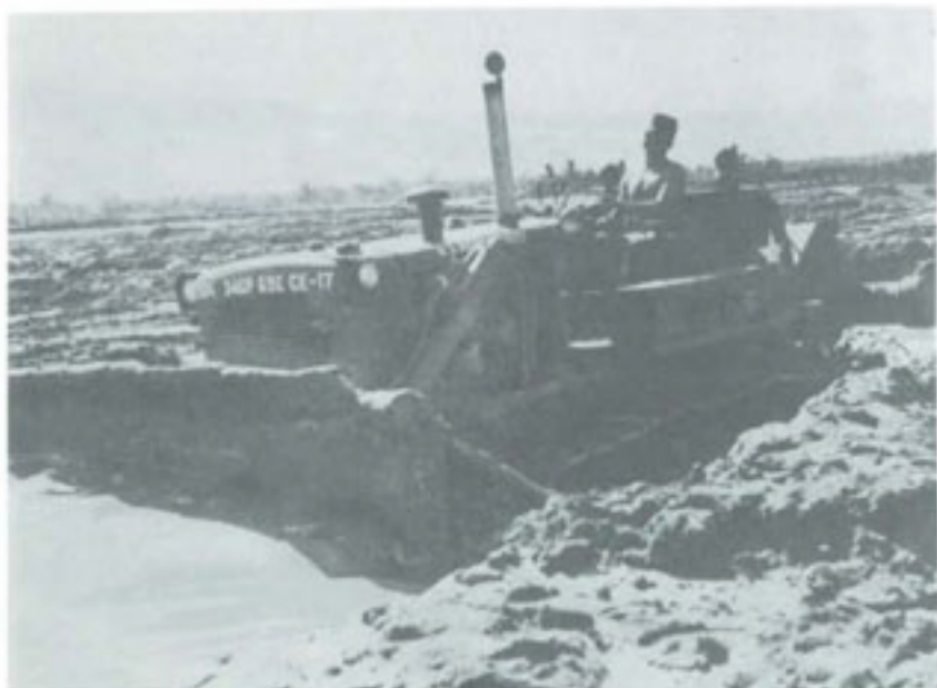
DOZER REDISTRIBUTES SAND DREDGED FROM RIVER
