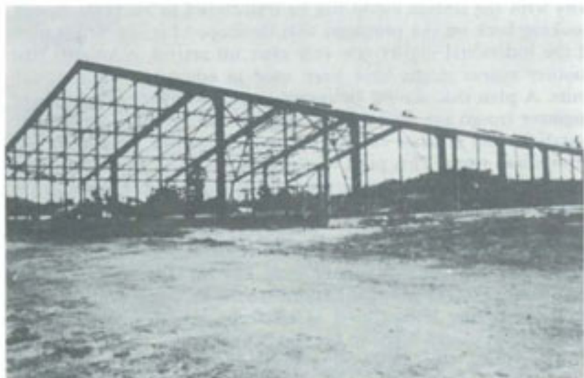
AIRCRAFT HANGAR UNDER CONSTRUCTION AT AN KHE
