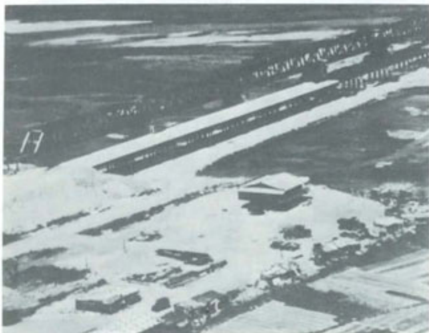
BRIDGE BUILT BY VIETNAMESE ENGINEERS NEAR TUY HOA
