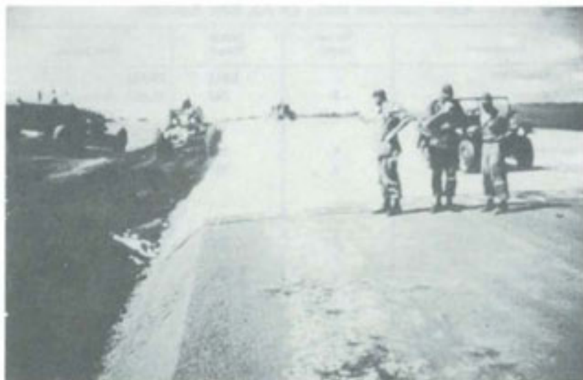
INSTALLING T17 MEMBRANE AT BAO LOC
