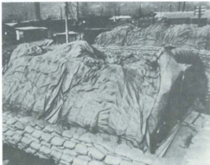
INFLATABLE HOSPITAL BUILDINGS AT DONG TAM DAMAGED BY MORTAR ROUNDS
