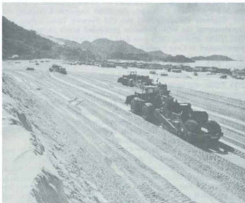
EARTHMOVERS LEVEL SAND at Cam Ranh engineer complex, 1965.
