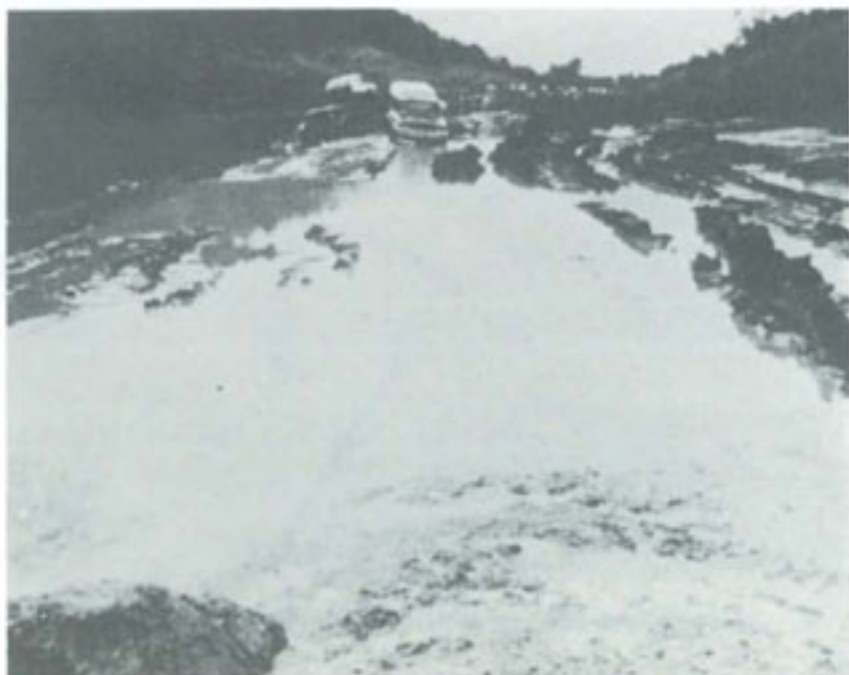
ROAD FAILURE IN THE DELTA
