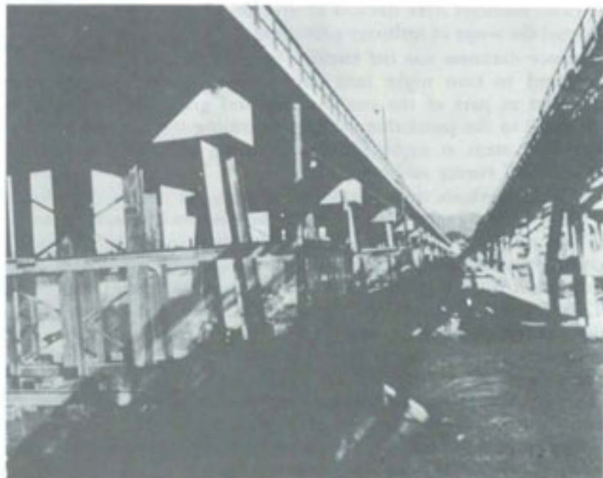
BRIDGE PROTECTED WITH CAGES AGAINST SABOTAGE on Highway 1 near Bong Son.
