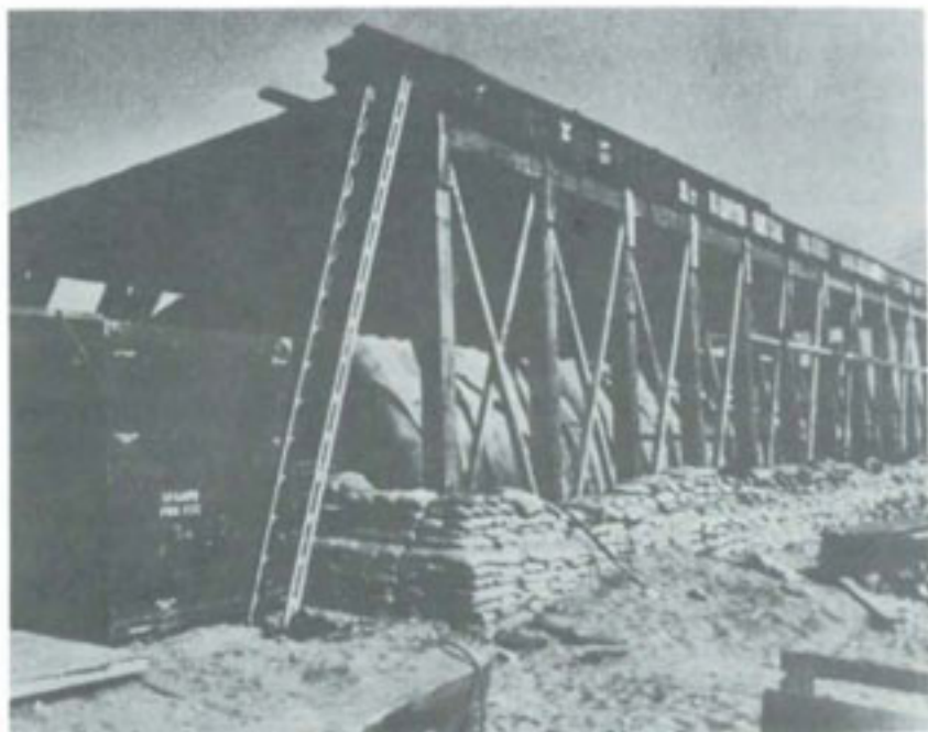
ENGINEERS' SHELTERS FOR INFLATABLE HOSPITAL STRUCTURES AT DONG TAM could withstand a direct hit by an 81-mm. mortar shell.
