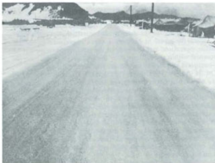
CRUSHED CORAL ROAD AT CAM RANH, built to test road building over unstable natural sands.
