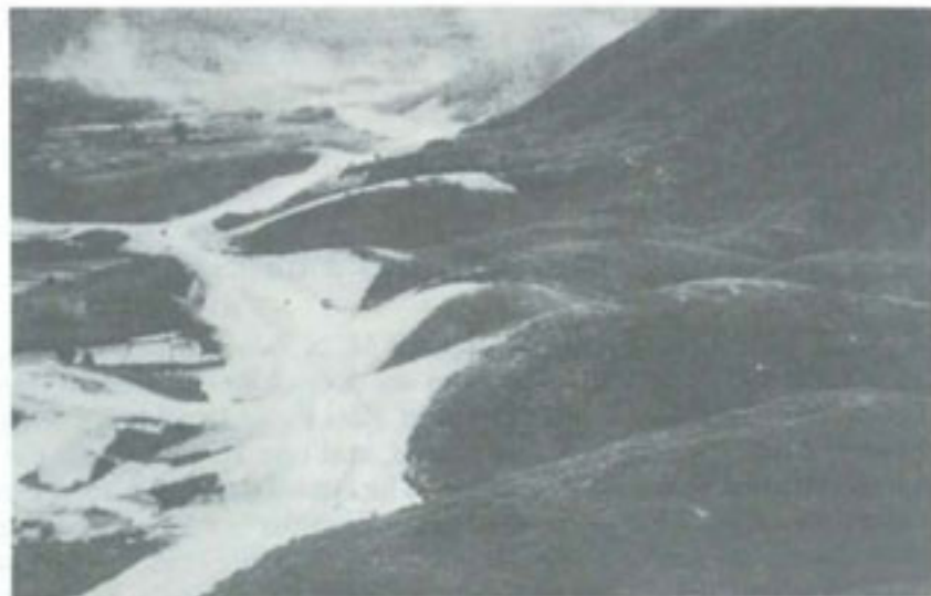
THE A SHAU EXPRESSWAY during upgrading by the 27th Engineer Battalion.
