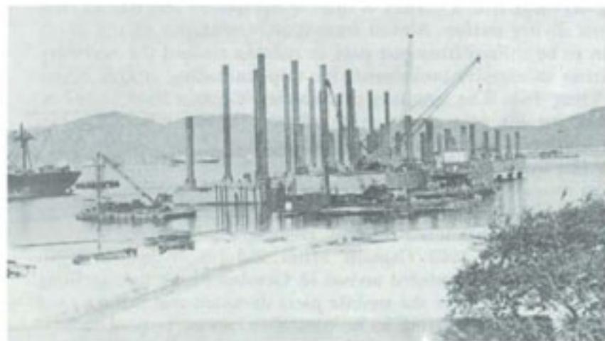
FIRST DeLONG PIER UNDER CONSTRUCTION AT CAM RANH
